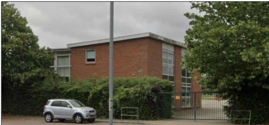
figure 72: Building Indicated as being Demolished
